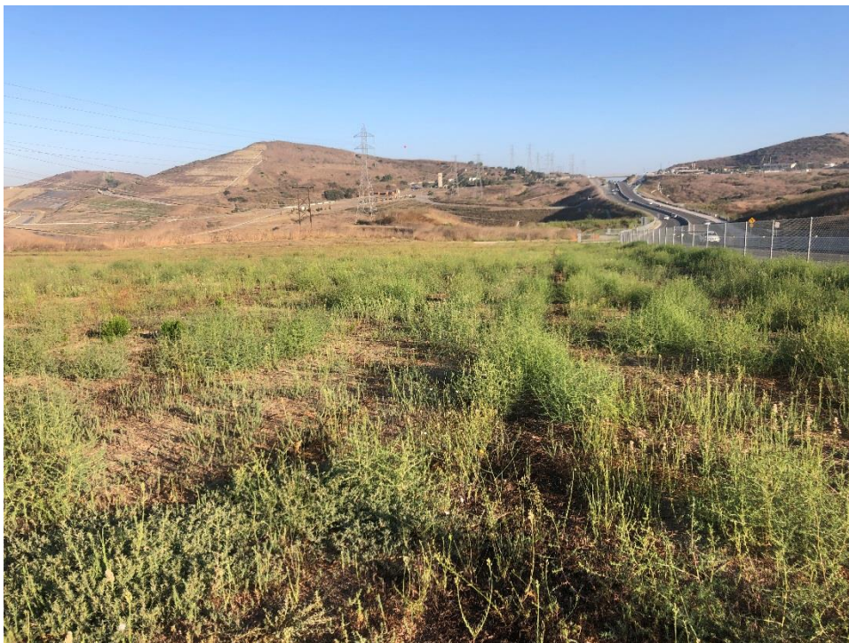
Photo 4: MPR-4 Western staging area location facing north
